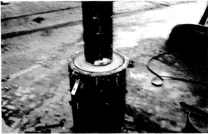
Figure 7. Refractory core casting method.
